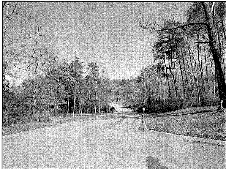
780 Woodlake Blvd Street
